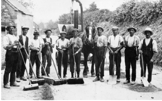
Local Authority road repair team at Pike Corner, 1922. Most of these men were from the village. Using watering cans, they applied hot tar to the road surface in patches and then sprinkled chippings on top.
