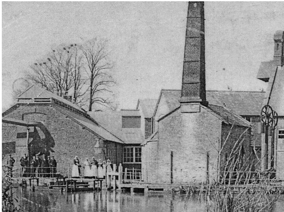
Tail Mill (circa 1900). Although the millpond is still evident, the tall chimney suggests that by this time a steam engine had been installed and that waterpower had been abandoned
