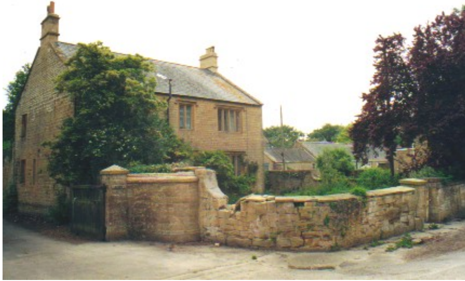
House in Merriott
