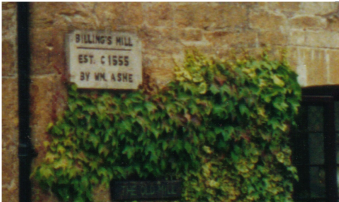
Close up of the Date Plate
